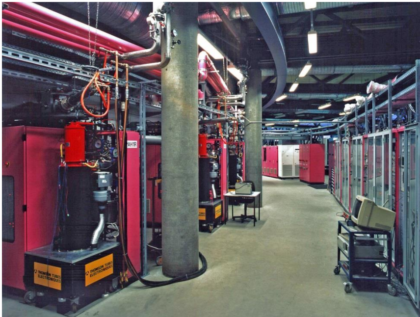
Old 75 kW 500 MHz klystron based RF transmitters
