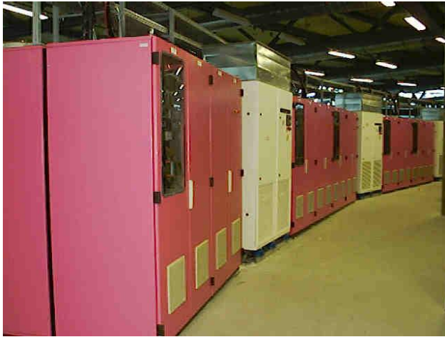
Old 75 kW 500 MHz klystron based RF transmitters
