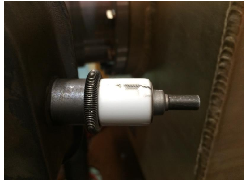
Connector of Klystron vacuum pump
