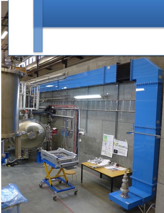
Waveguides by EXIR are installed in FREIA
